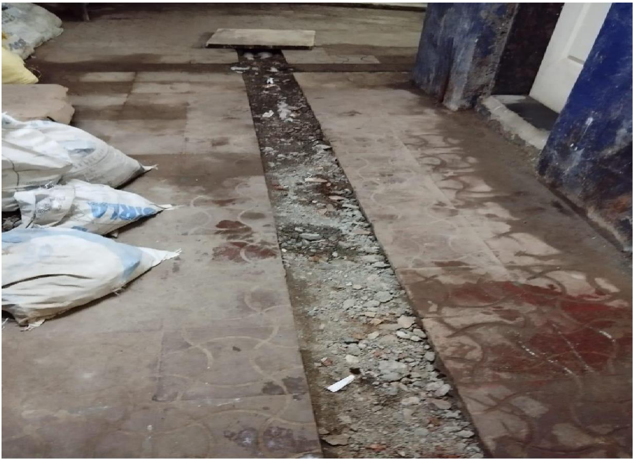
Image 4: Washroom in the Malabar Hill Police Station
