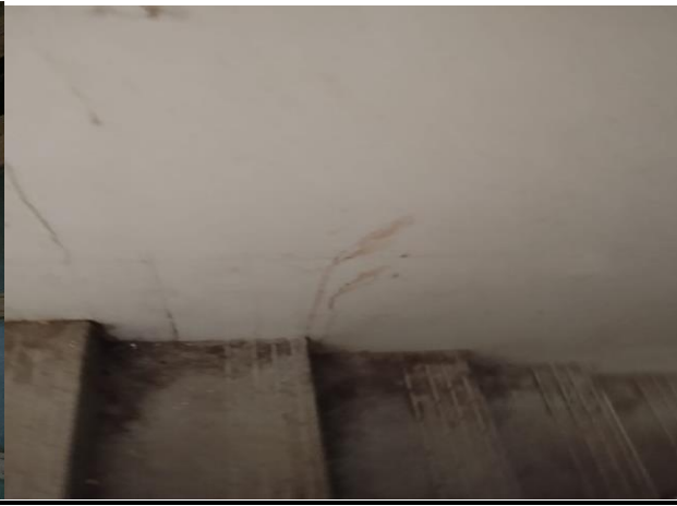
Image 3 : Stairs at the Police Station
